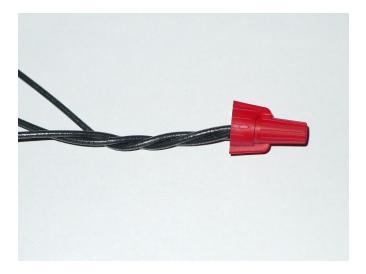
Repeat with the 3 red tips from the Fan, Pump, and Extension wire.
